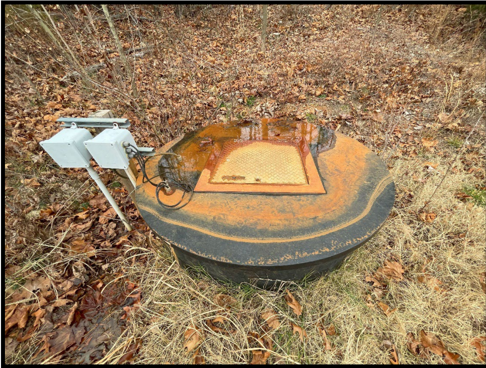
Photograph 1: View of VLCS-1 at capacity and beginning to overflow.
